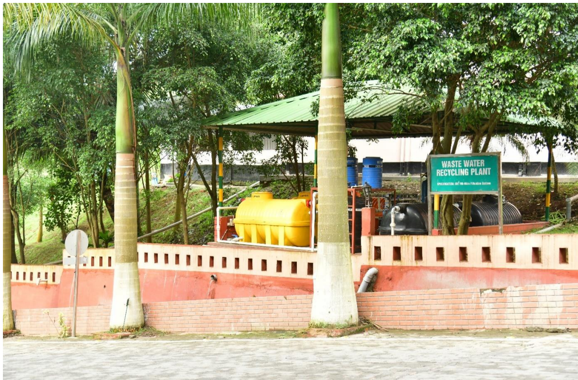
Waste Water Recycling Plant
