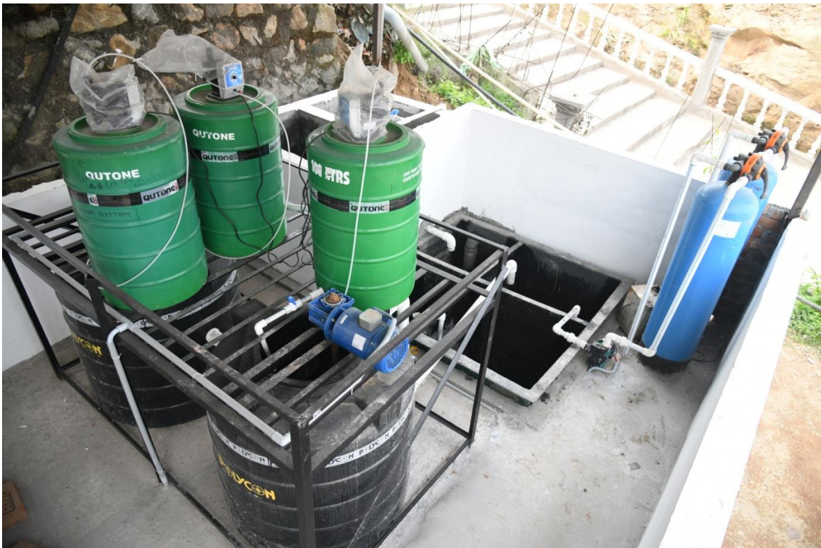
EFFULENT TREATMENT PLANT
