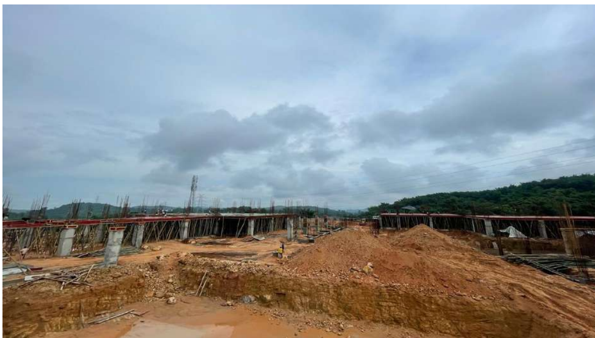
Construction Site of PA Sangma international Medical College & Hospital
