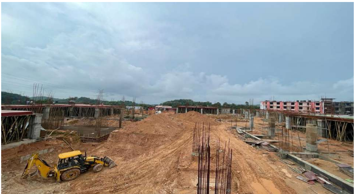
Construction Site of PA Sangma international Medical College & Hospital
